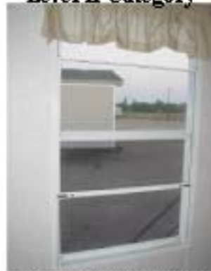
Windows with Storms
