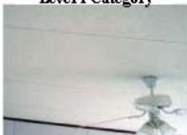
Pre-finished Ceiling Boards with Seams
